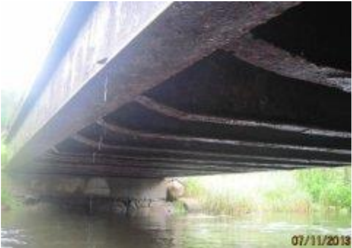
Bridge No. 35; Note extensive rust.
