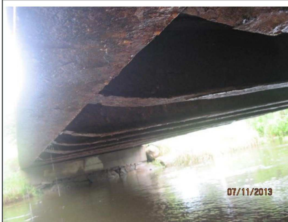
Figure 3. Floor beams noted as crushed in the July 2013 inspection report
